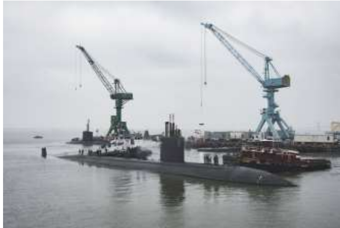
The attack submarine Boise arrives at Huntington Ingalls Industries' Newport News, Va., shipyard on June 18, 2018, to begin an extended engineering overhaul.
